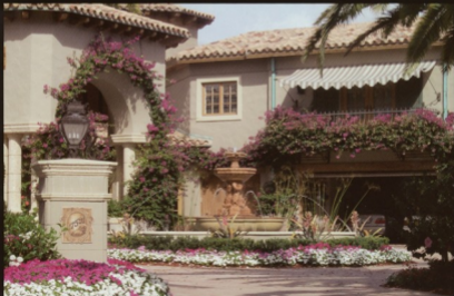
Bougainvillea entwined with Mediterranean architecture frames a hand-carved fountain which provides the focal point for this St. Andrews estate in Boca Raton, Florida. General contractor: Weitz Construction. Image provided by Krent Wieland Design, Inc.
